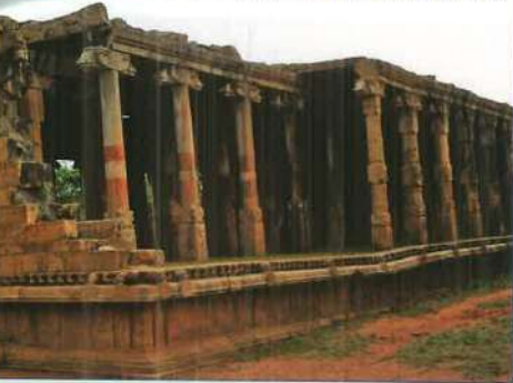
Chariot structure - Kunnandar koil (Hundred pillar hall)
