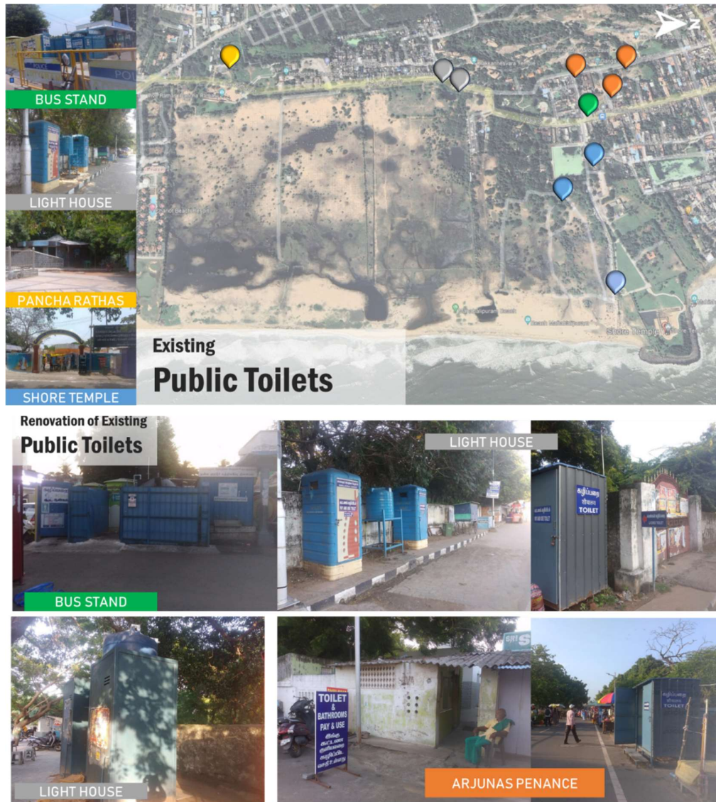
Figure 6-19 Location & condition of Existing Public Toilets
