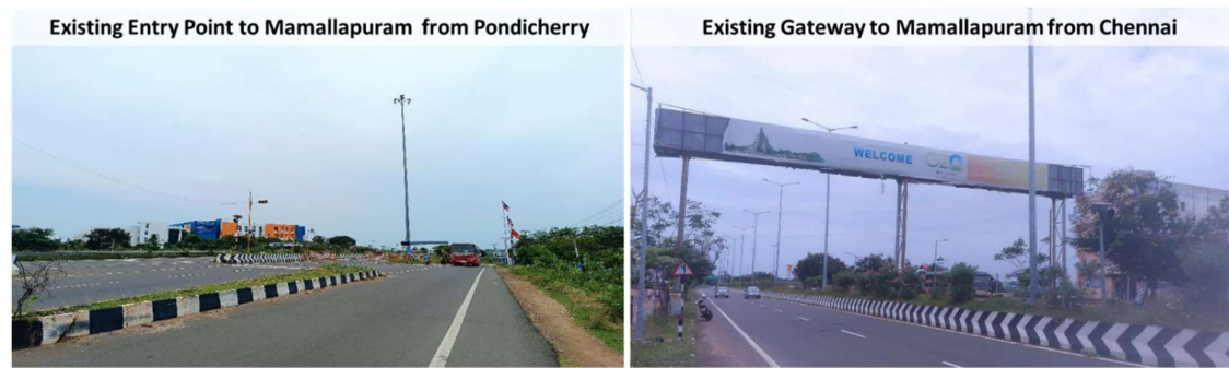
Figure 6-3 Existing situation of the identified entrance arch/gateway areas
