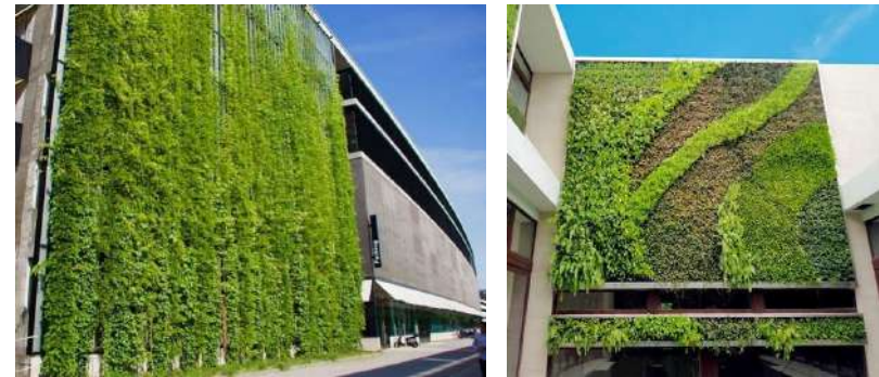
Creeper Walls for site boundary
