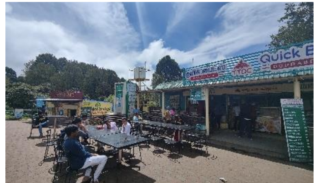
Water ATM not functioning, and the food court doesn't have a roof shade.
