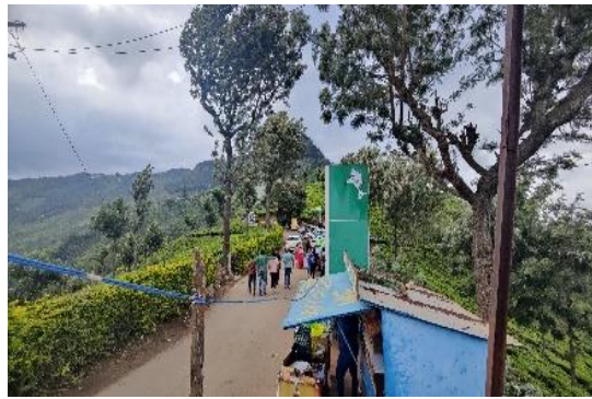
The walkway to the destination area is not sufficient and the shops on the road side are not in a proper condition
